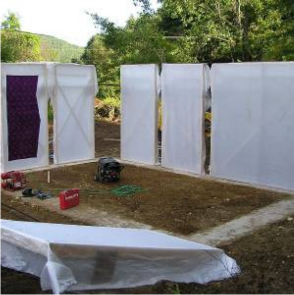
Fig. 4. Wall Form Placement
