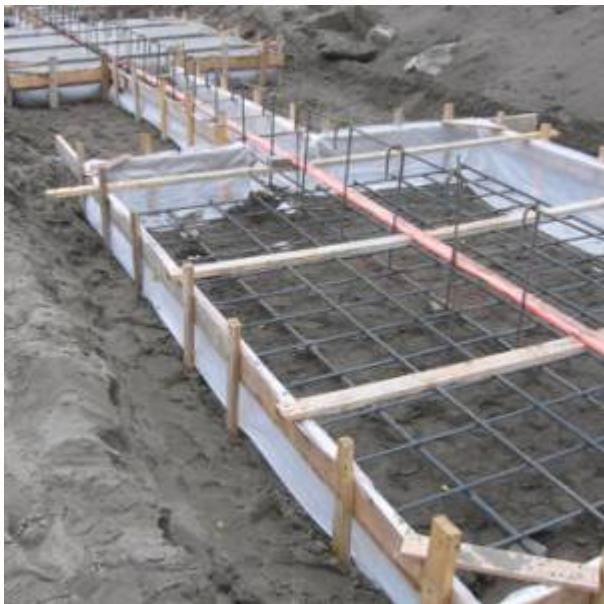
Fig. 1. Spread/Continuous Footing Application
