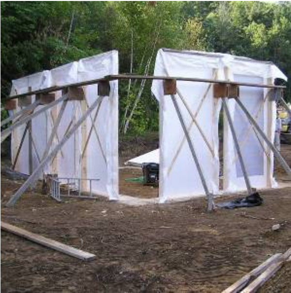
Fig. 5. Wall Form Placement
