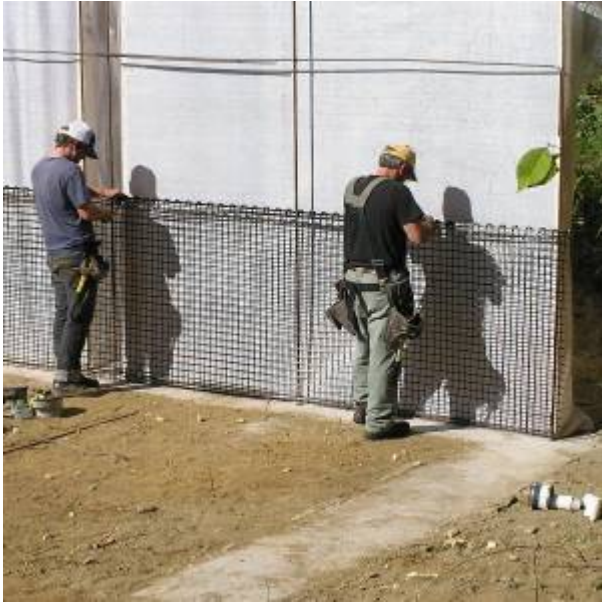
Fig. 6. Adding Carbon Fiber Grid
