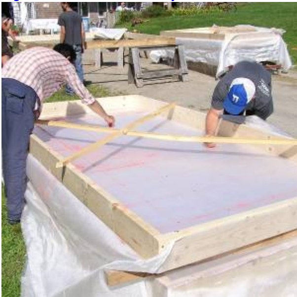
Fig. 3. Wall Form Assembly
