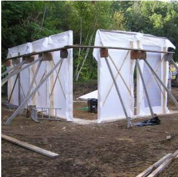
Fig. 5. Wall Form Placement
