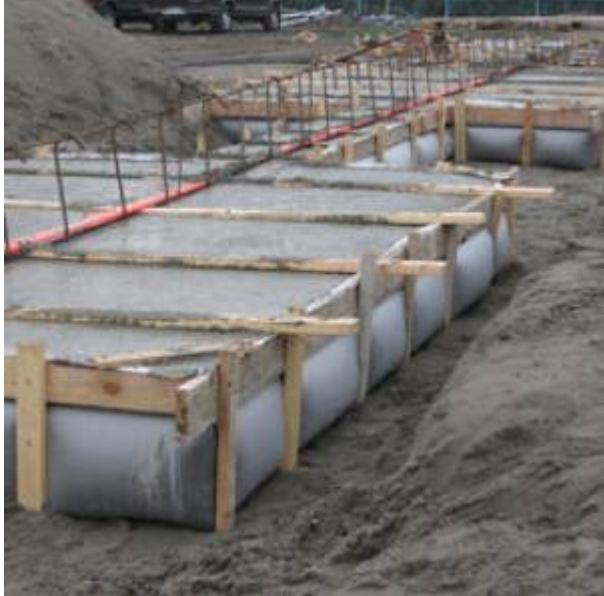
Fig. 2. Spread/Continuous Footing Application
