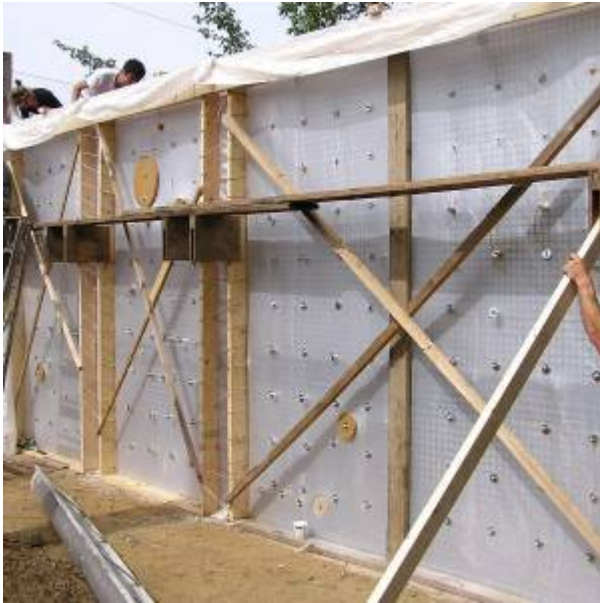
Fig. 8. Wall Form Placement
