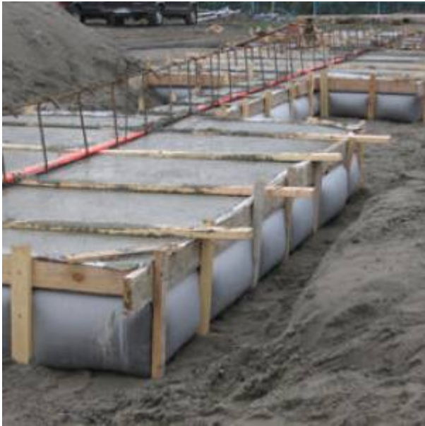
Fig. 2. Spread/Continuous Footing Application
