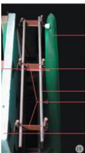
Fig. 18 illustrates Unno's Zero-Waste Formwork Membrane (in this case scaffold membrane could also be a re-usable polycarbonate). This Membrane would be restrained "frame" or "quilt-point" methods (not shown in image) as described earlier. Removal of the Membrane leaves a beautiful exposed concrete surface and thermal mass to the interior.
