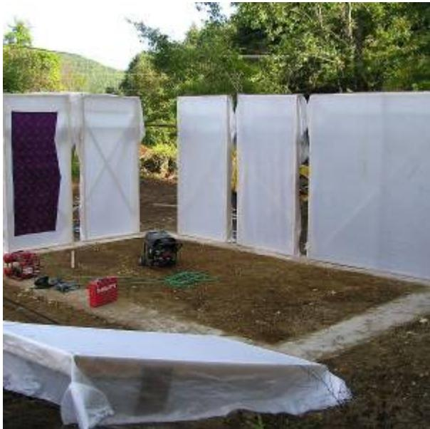
Fig. 4. Wall Form Placement
