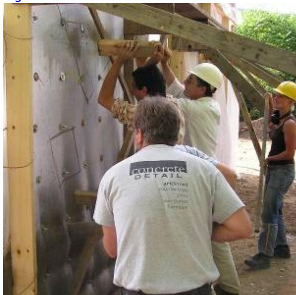
Fig. 11. "Vibrating"Concrete
