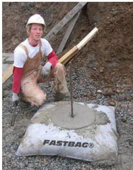
Fig. 3. Spread Footing Application
