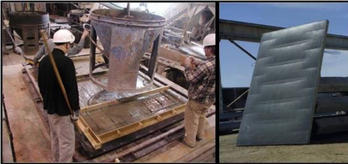
Fig. 1. Full-scale formwork and completed concrete panel.
