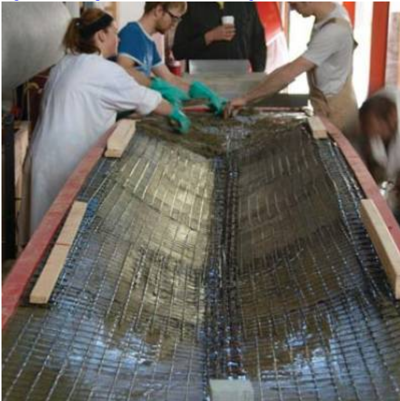
Fig. 40. Placing concrete and carbon grid (Portland cement mortar mix used) for...
