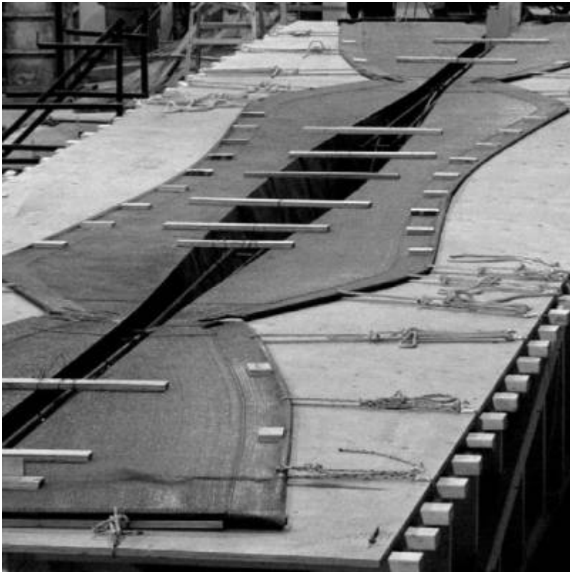
Fig. 11. Plywood deck and fabric formwork for variable section beam.
