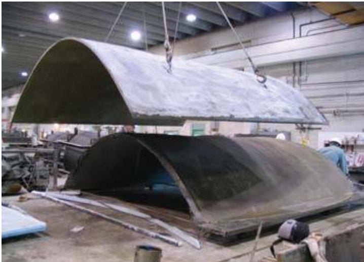
Fig. 23. Step 2- Uniform layer of GFRC is applied.
