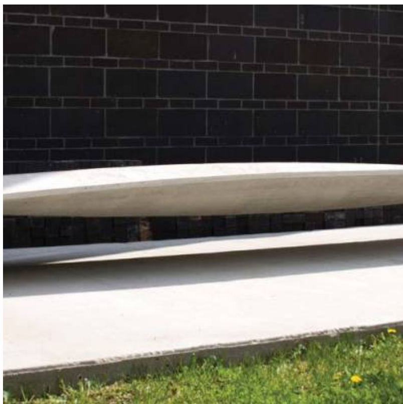
Fig. 41. Completed double-curvature lenticular thin-shell vault.
