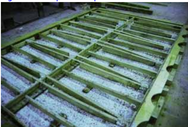
Fig. 9. Formwork for full scale wall panel.
