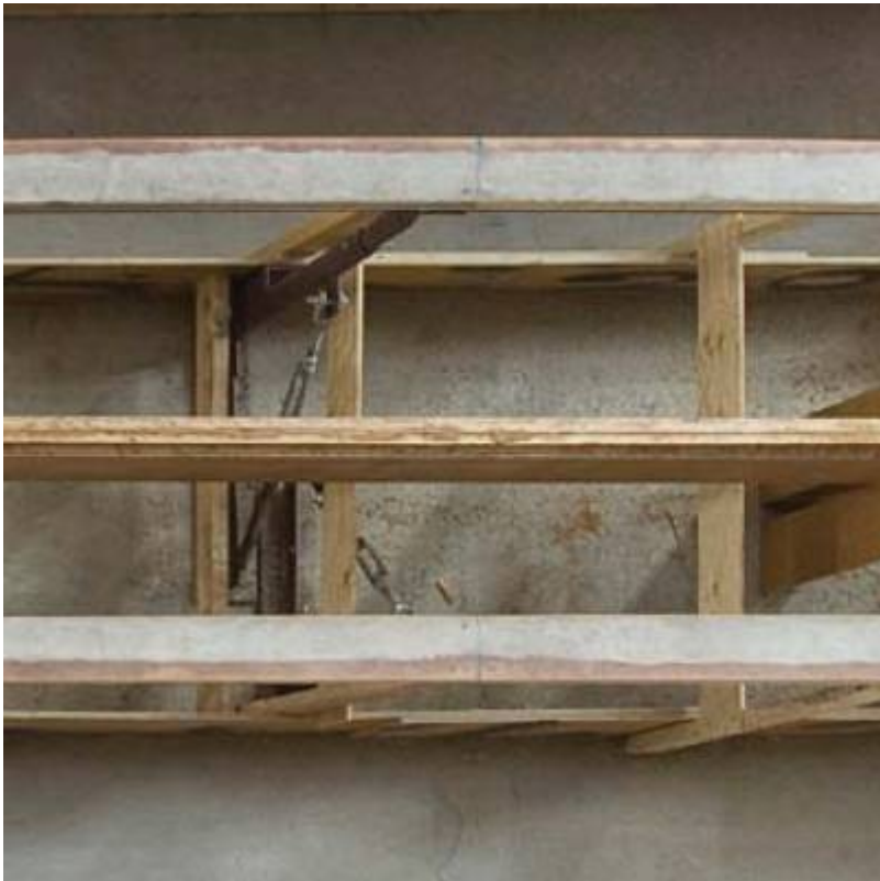
Fig. 37. Perimeter frame with "keel" on which fabric is hung.
