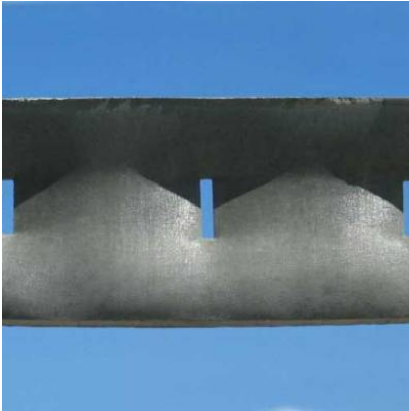
Fig. 9. Close up view of completed full scale variable section concrete...
