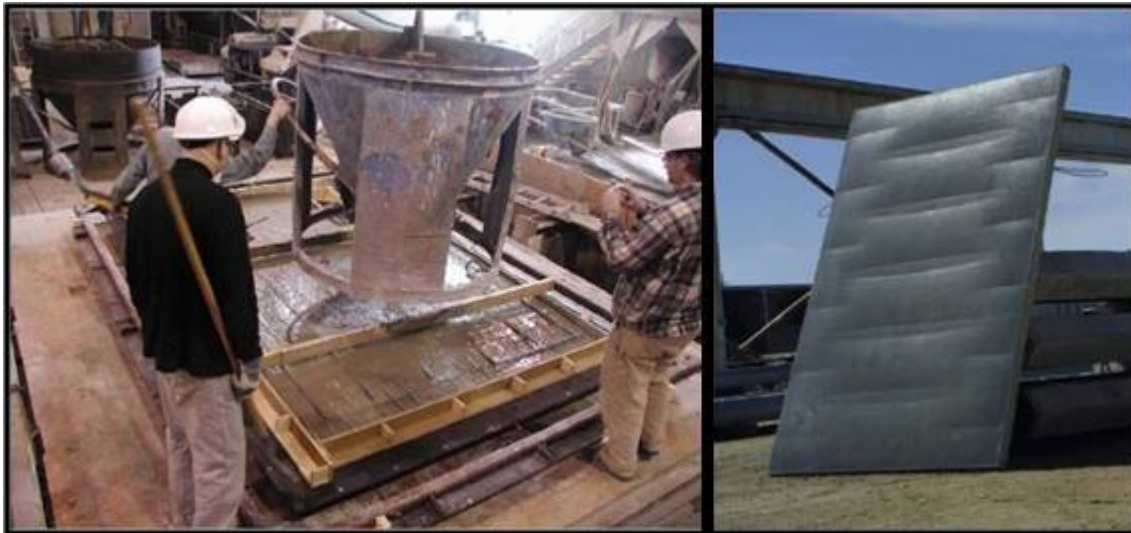
Fig. 2. Full-scale formwork and completed concrete panel.
