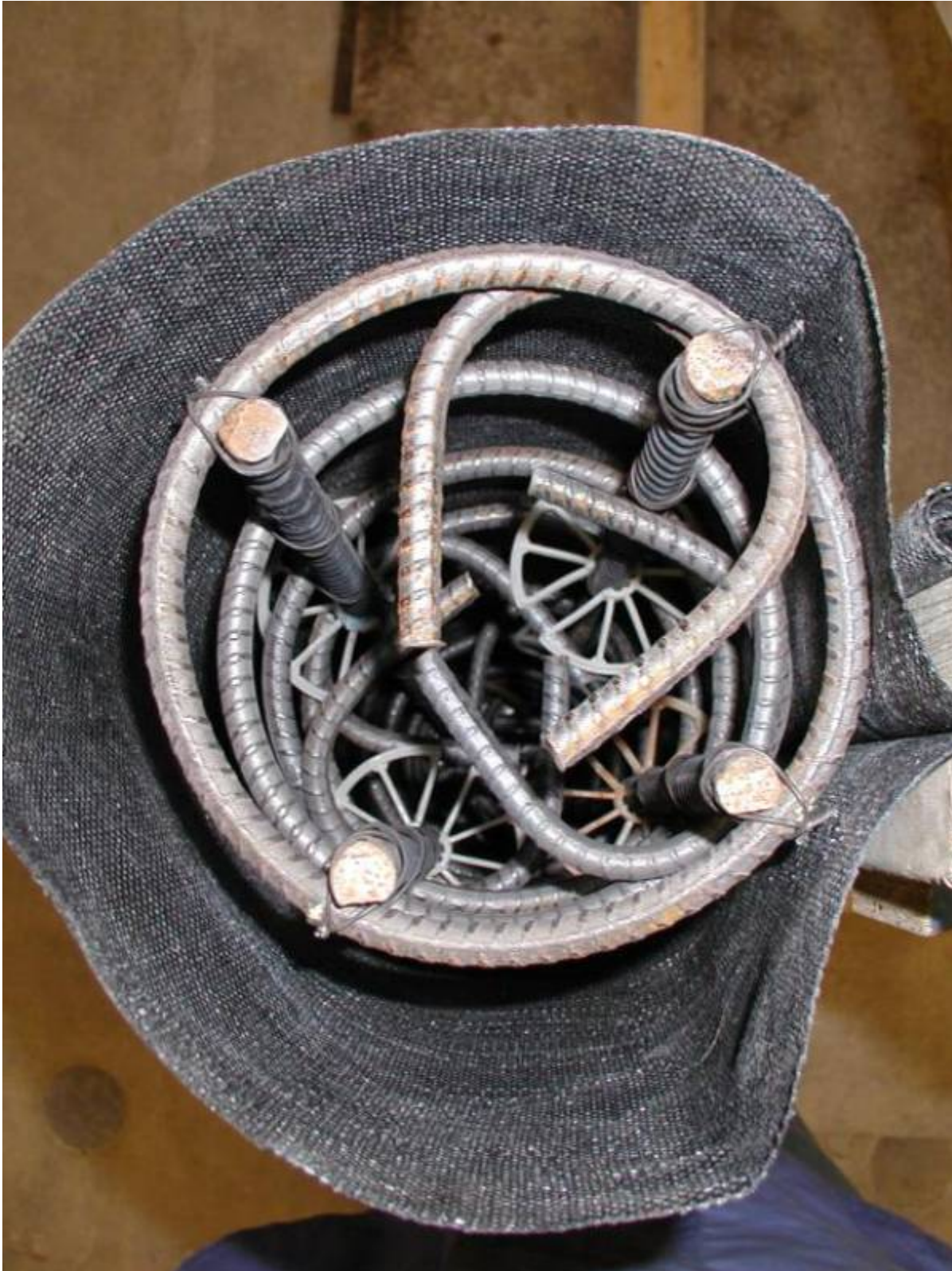
Figure 46: Reinforcement cage.
