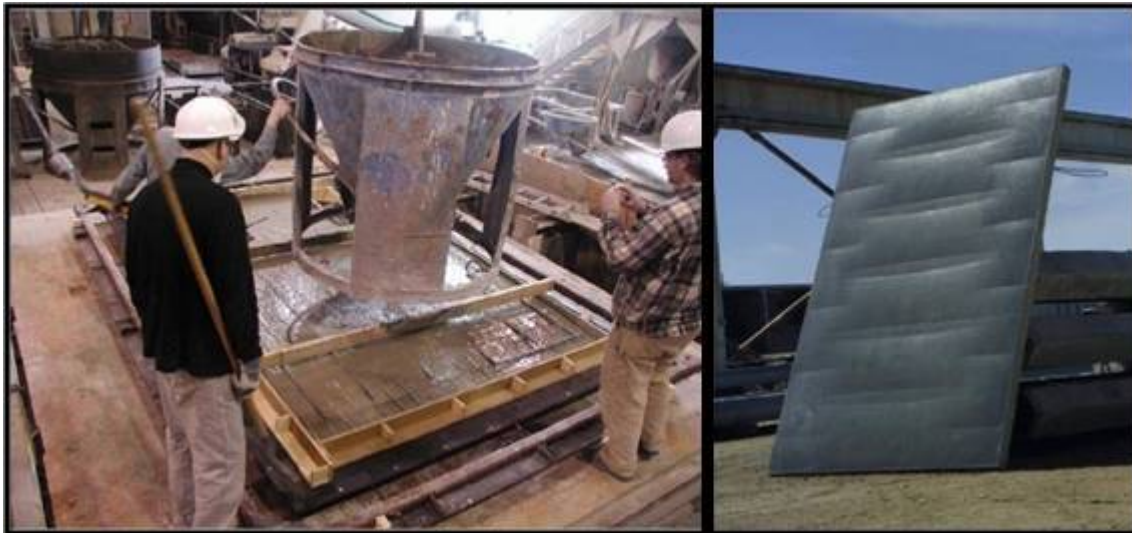
Fig. 2. Full-scale formwork and completed concrete panel.
