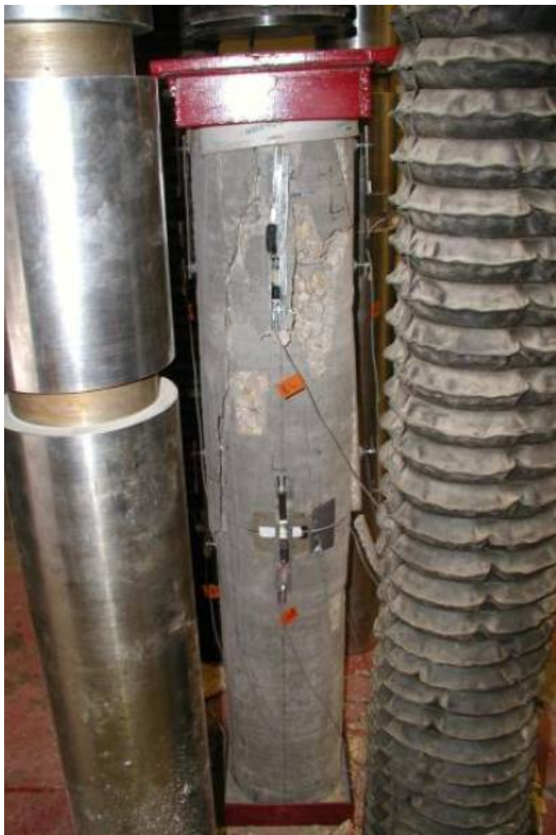
Figure 65: Column FF-FAC after failure.
