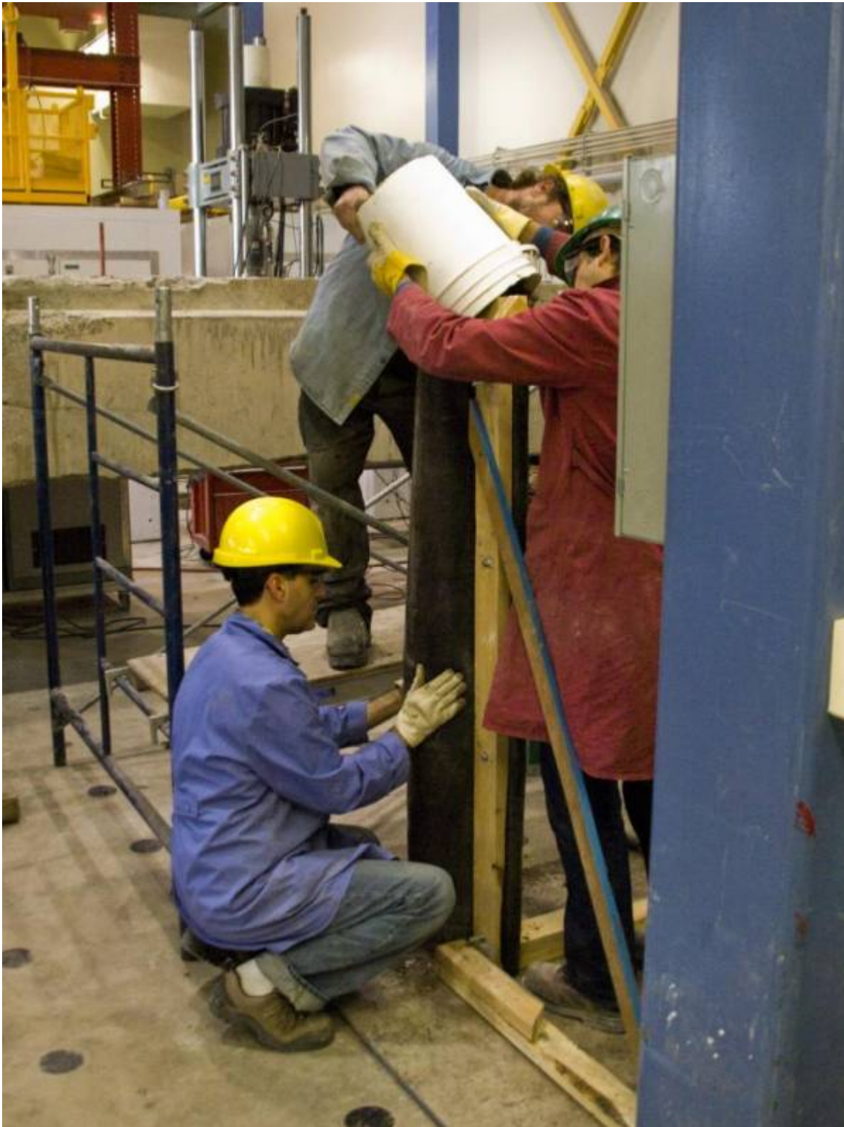
Figure 47: casting of column in fabric formwork.
