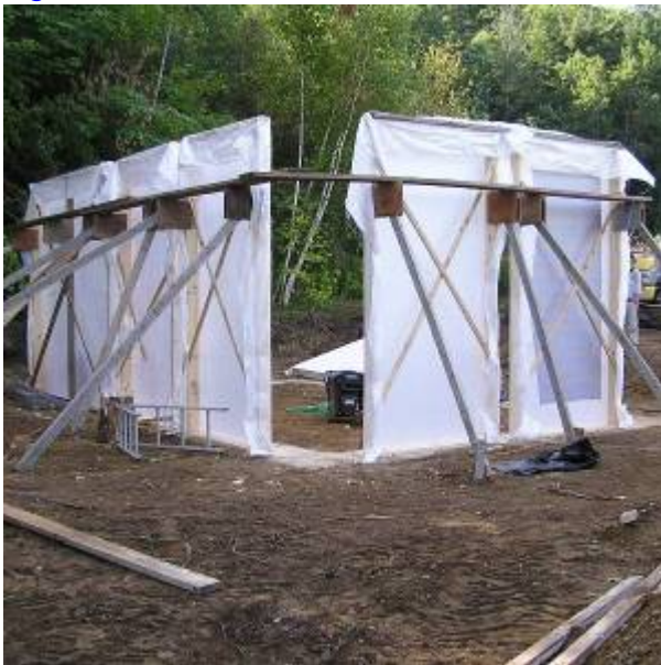
Fig. 5. Wall Form Placement
