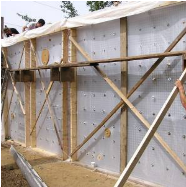
Fig. 8. Wall Form Placement
