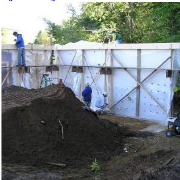
Fig. 7. Wall Form Placement
