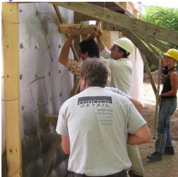
Fig. 11. "Vibrating" Concrete
