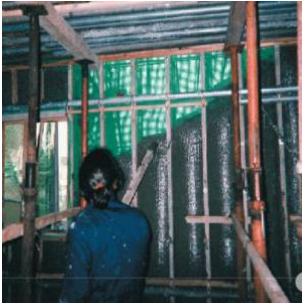
Fig. 1. Frame Form Method
