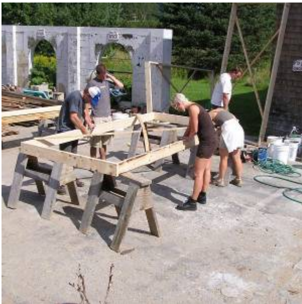
Fig. 1. Wall Form Assembly
