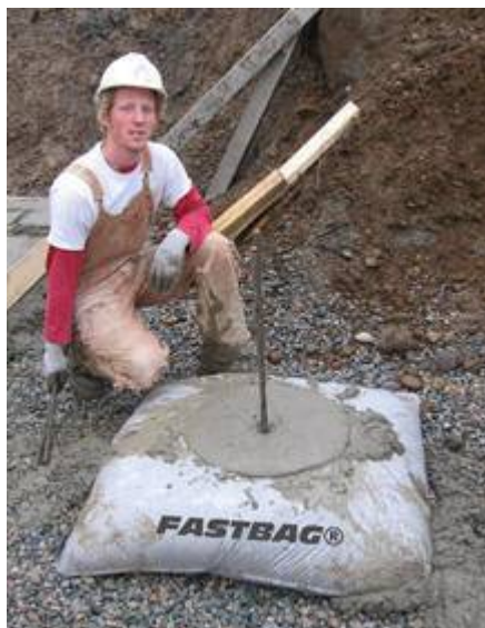
Fig. 3. Spread Footing Application
