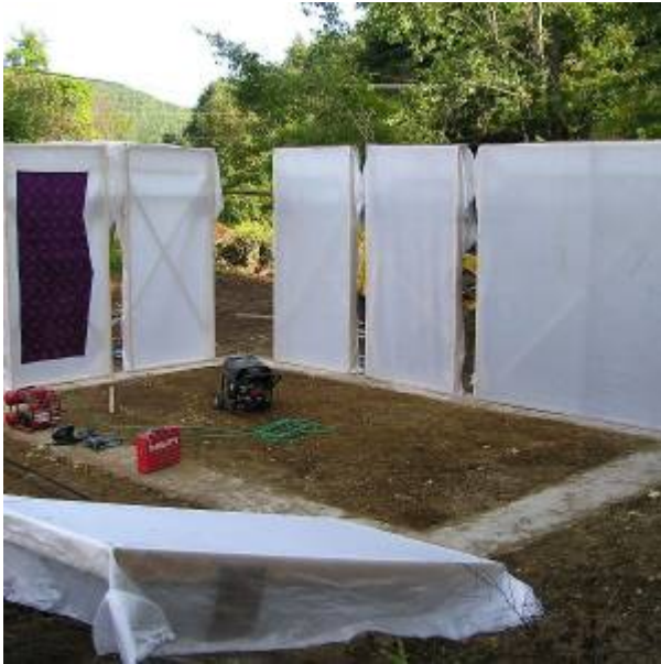
Fig. 4. Wall Form Placement
