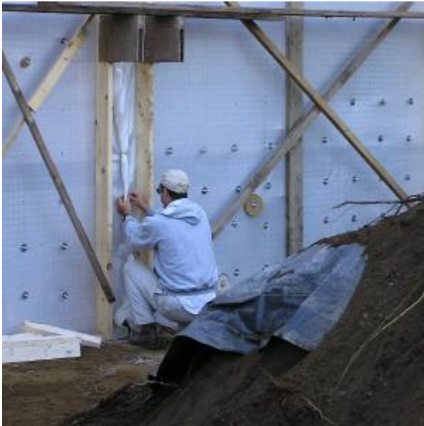
Fig. 7. Wall Form Placement
