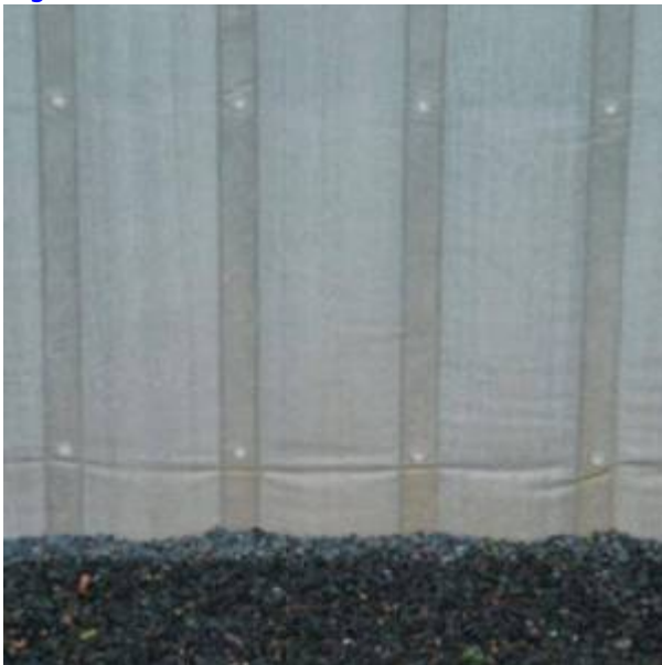
Fig. 2. Frame Form Method
